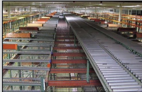
VIEW OF MEZZANINE
